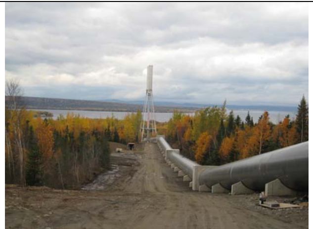
Completed project with steel penstock and refurbished surge tank.
