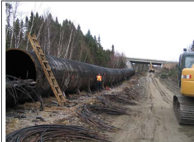
Creosote woodstave penstock being removed during construction.
