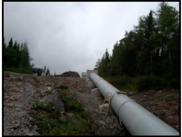
Lockston Penstock after installation of steel penstock
